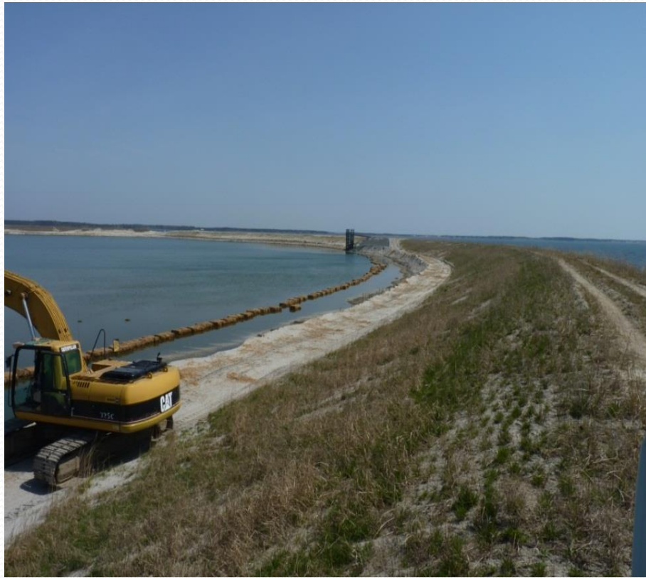
Newly Planted Berm Vegetation
