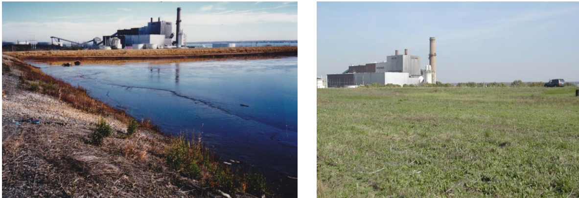
Figure 3. Site #2 DuPont Edgemore Titanium Dioxide Sludge Disposal Containment, i.e., Final Cover
