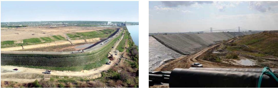
Figure 2. Site #1 Delaware Solid Waste Cherry Island Landfill Containment Wall
